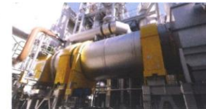
② 汚泥乾燥機(攪拌機付き回転キルン) Sludge dryer (rotating kiln with mixer) 熱風温度を約 580℃に調整しながら下水汚泥を水分 10%~30%となるまで1時間程度乾燥させます。 Sewage sludge is dried for about 1 hour/units until its moisture content becomes 10 to 30% while the hot air temperature is adjusted to about 580°C.
